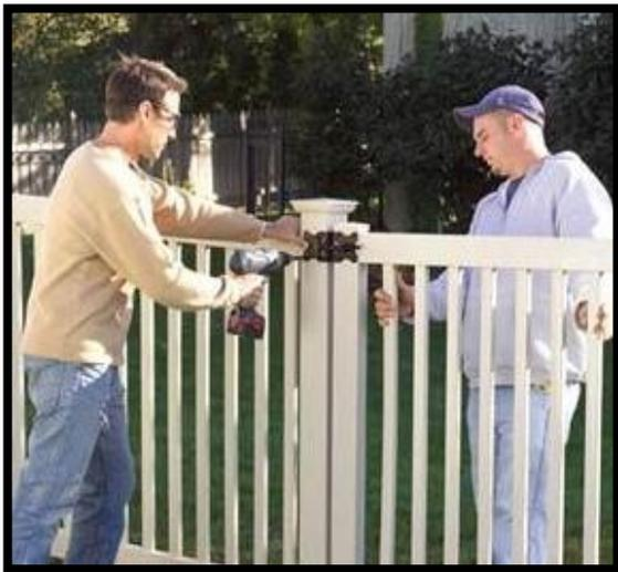
Hang the gate- Screw the hinges and latch to the gate. Then center the gate in the opening and screw a catch to the other post.
