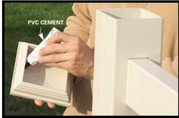
Cement Caps- Add a small dollop of PVC cement or silicone caulk to the tabs at the top of each cap and push the caps over each post.
