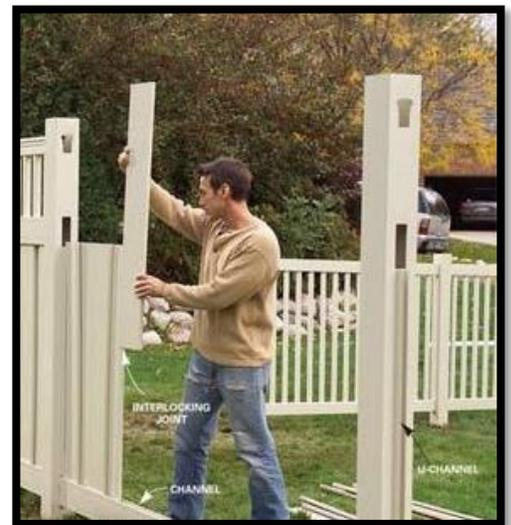
Position Boards- Slide the interlocking vinyl boards into the channel in the bottom rail. Screw to the U-channel.
