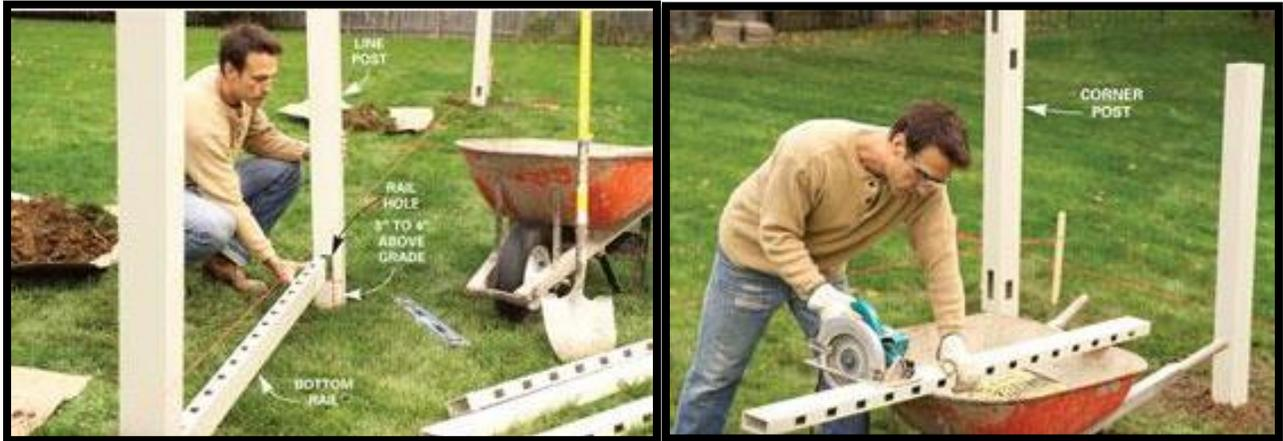
Plumb Post- Drop a post into place and snap in the bottom rail. Then position it against the string line, Plumb it and add concrete.
