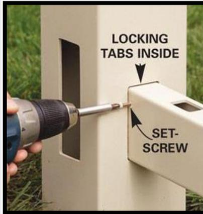
Lock Rail- After aligning the post, lock the rails in place.
