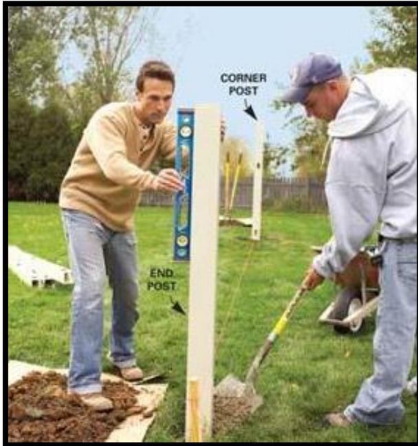
Layout the Fence – Stretch a string line tightly along the proposed fence run, locate the corner posts and dig 3-ft. deep postholes. Plumb the post and fill the holes with concrete.
