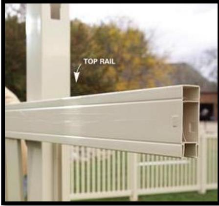
Slide the top rail over the boards, locking the end into the rail hole, and then into the rail hole at the opposite end.
