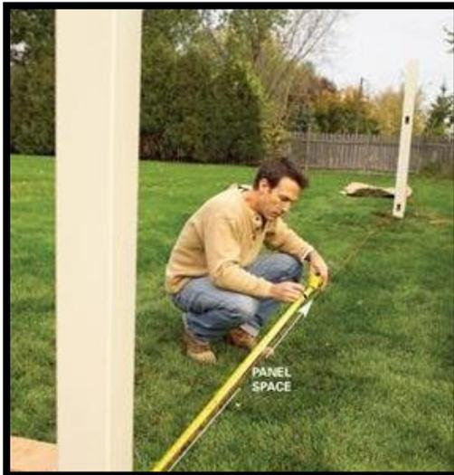
Locate Post- Mark the post location on the line and then march each posthole with a stake.
