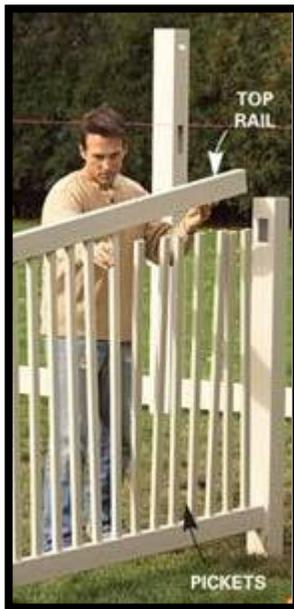
Add Pickets- Slip pickets into the bottom rail. Snap the top rail into one post, slip it over the picket tops and snap it into the other post.
