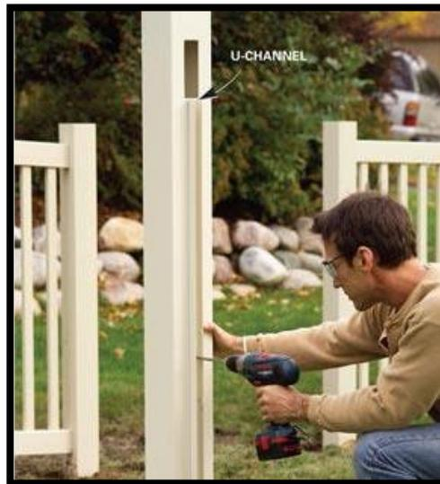
Fasten U-channels- Center and screw U-channels with three evenly spaced screws into fence post for privacy panels.
