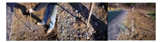
Post preparation is strongly suggested. We like to cut a small triangle out of one corner of the post about 8 - 10 inches from the bottom to give the concrete a place to 'grab'. A couple of the self-drilling screws are an alternative to consider. This point also serves as
