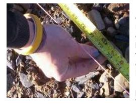
Post spacing is measured from center of post to center of post. The correct center to center measurement for OnGuard residential grade pool code fence is 72-1/2 inches and this varies from brand to brand. If there is no building to work from, we start at the location of a gate post or an end/corner. We locate the holes along the string line using a nail to designate the center remembering that we are marking the center of the post and taking that into account when placing our first nail.
