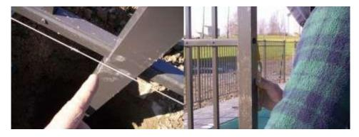
We maintain the 1/16 of an inch gap between the post and the string and constantly check the plumb of the post.
