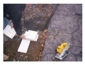
When it's time to install the section we lay out 'spacers' to support the bottom rail and keep the correct clearance from the grade. We use pieces of vinyl fence pickets close to or right at the post. 2x4's or 1x4's work just the same. We keep our eye on where the post is at on the string. Even the best installers can mistakenly throw the line off. On level ground, we can sometimes get 3 or 4 sections ready to be poured at one time.
