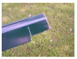
We often make our marks using a square and an awl or similar tool to scratch the finish; a pencil line may be hard to see on dark material. You may notice that the cut is not exactly on the mark; this allows it to be inside the post where it won't be seen.
