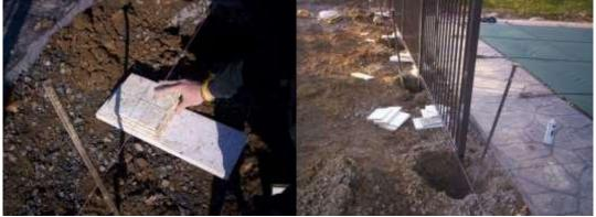
If we 'top' the holes the same day or not, we continue to lay out our spacers and install the sections maintaining the same 1/16 of an inch gap between the post and the string. We move our digging bars from those posts where the concrete has set sufficiently and work toward the corner.
