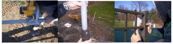
As mentioned previously, loose dirt should never be put back in the hole. This may be a tempting solution if you think you've dug too deep and want to save on concrete. Installation longevity comes from proper post depth so we *purposely* over-dig and drain the posts with a piece of PVC. 1-1/2 inch pipe or electrical conduit is dropped into the post *before* inserting the rail ends. We prefer this method over a 'weep hole' drilled in the post right at grade.
