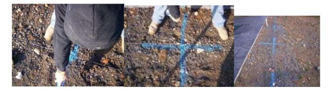
When we are going to use a machine to dig the holes, a large X will help us get back on track if we hit rock and the bit 'wanders'. A small mark will be obliterated as soon as we start to dig. The line that is painted parallel to the string should be 1 inch away from it
