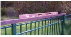
If the installation requires that the fence is level as opposed to following the grade, we find it more effective to use a post from post top to post top and place the level on it rather than on the rail of the section itself. This is especially important when using a short level. The rails might become slightly distorted while the section is sitting on spacers located closer to
