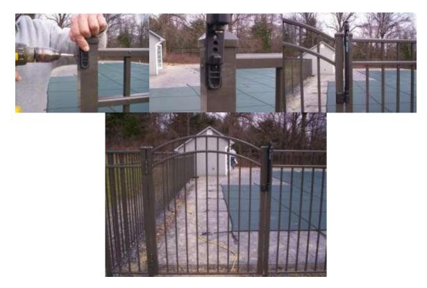
After we've installed the Magna latch according to the instructions provided by the manufacturer we go back and install the post caps checking first to be sure we've screwed the sections together as previously described. We install the caps with the 'heel' of our hand. When installing gate caps on the latch side we like to support the bottom of the gate.
