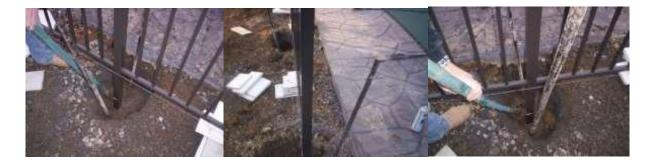
We use digging bars in the hole alongside the posts to hold them as the concrete is poured. It is advisable to 'poke' the concrete to eliminate any air pockets. We pay
